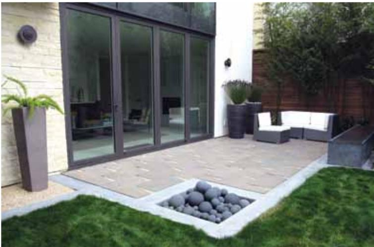
The patio features custom permeable limestone pavers with little triangles cut out. To allow water to pass through, the pavers were set on sand and the triangular spaces filled with gravel. “The patio has a nice graphic pattern when viewed from the floors above,” Haugeland says.
